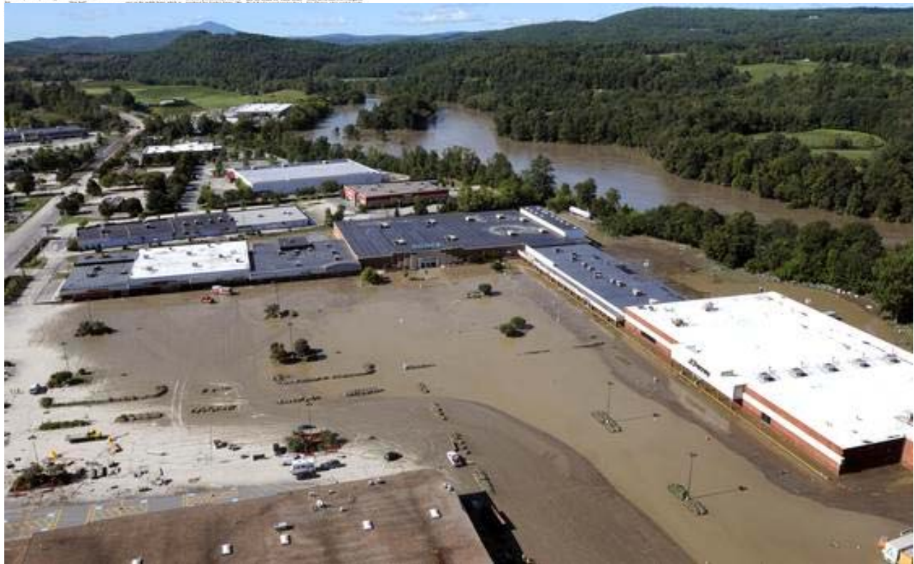
FLOODWATERS FROM TROPICAL STORM IRENE WERE STARTING TO RECEDE AT UPPER VALLEY PLAZA ON ROUTE 12A IN WEST LEBANON. (VALLEY NEWS — JENNIFER HAUCK) HTTP://WWW.VNEWS.COM/08302011/8007536.HTM
