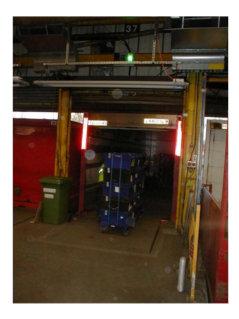
Figure 2: Dock door with RFID reader and indicator lights.
